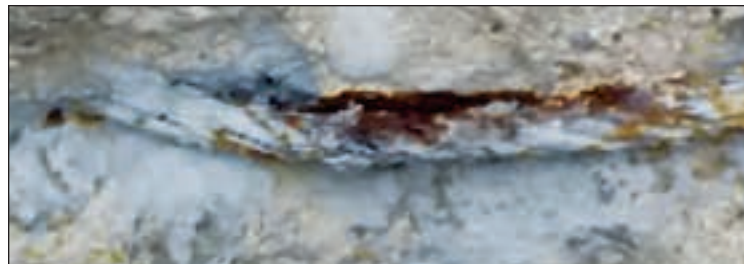
Cable "rebar" was used in the Bucoda Community Center when it was built.
